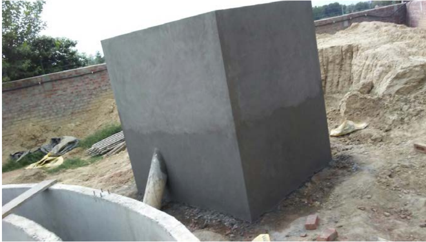
SLURRY FEEDING TANK
